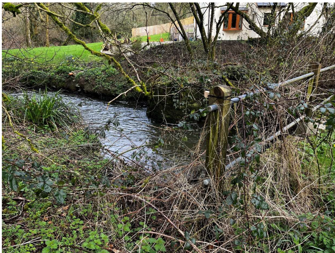
Plate 4-1 Photograph of posts at Rudbaxton Bridge on 21 March 2024
