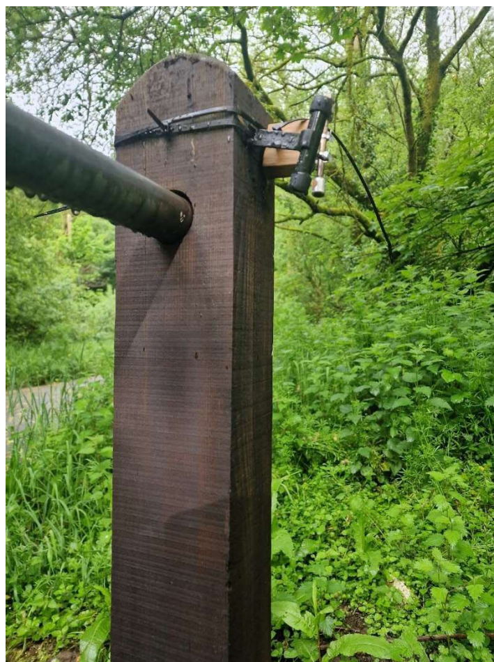
Plate 4-2 Photograph of posts at Rudbaxton Bridge on 16 May 2024
