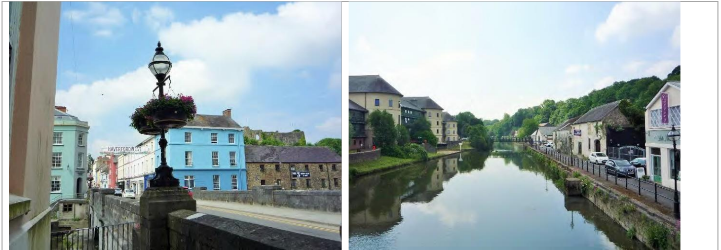
Gateway into Haverfordwest historic centre over Western Cleddau bridge and the urban river corridor
